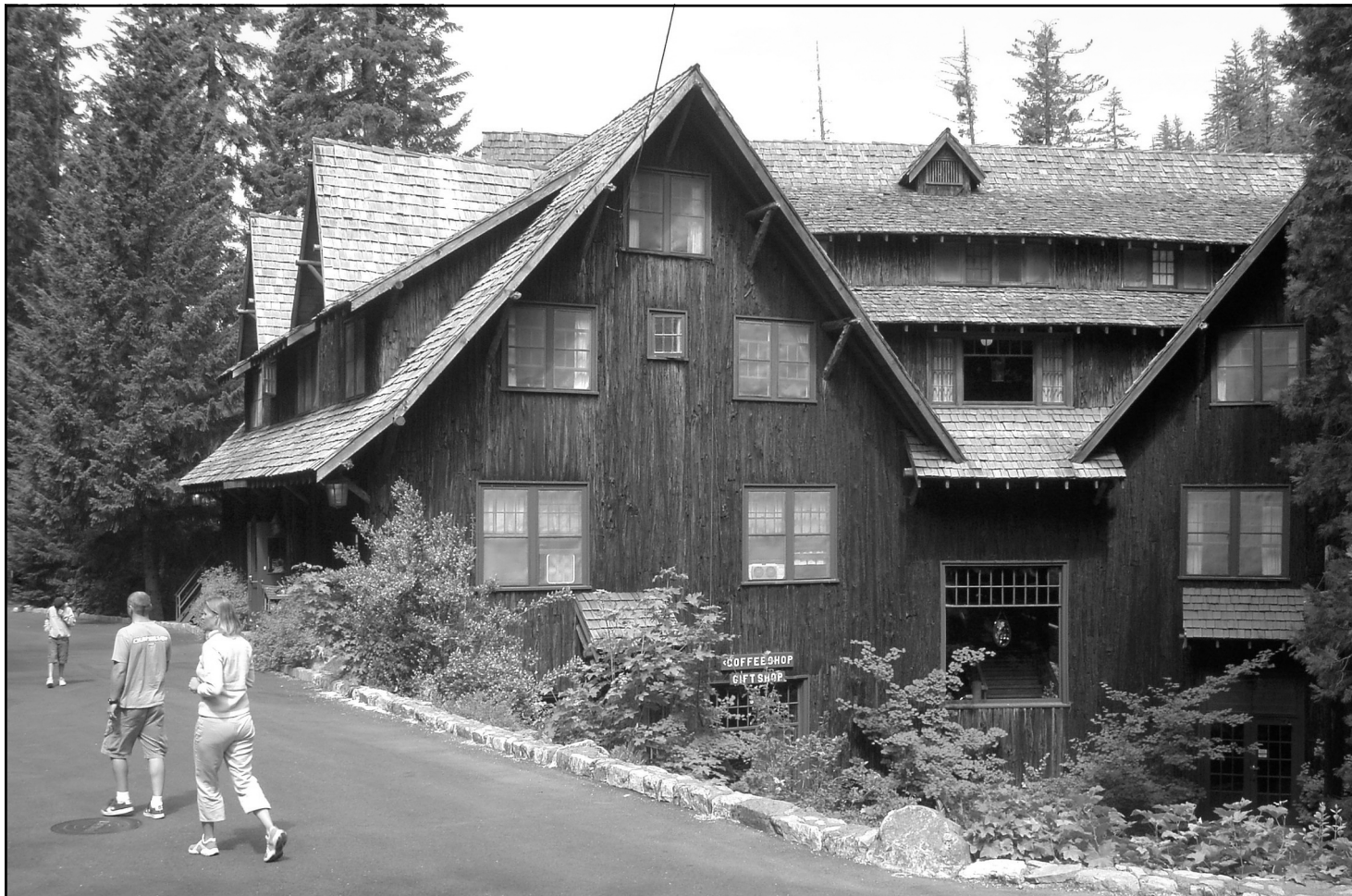
HISTORICAL CHATEAU - Illinois Valley attractions include the historic, rustic Chateau at Oregon Cave National Monument, some 20 miles east of Downtown Cave Junction. The building, which some call the 'Lodge,' has 26 rooms for lodging guests. The impos-
