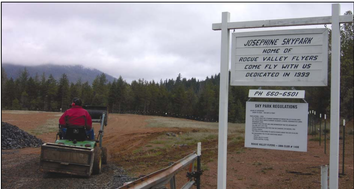
NEW AIRFIELD IN KERBY - Members of Rogue Valley Flyers were working on Sunday, April 27 at the former Kerby landfill at the end of Kerby Mainline Road, continuing their work on an airfield for radio-controlled model aircraft. The club has been working since 1999 and the site is now open for member pilots. Also the public can watch flyers. (Related photo on page 11)
