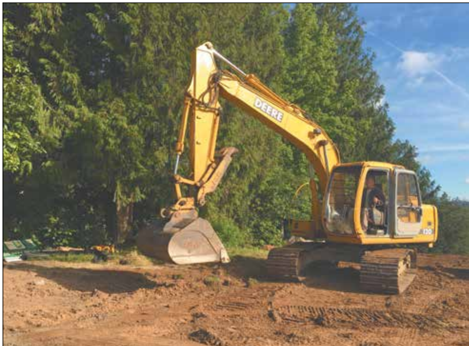
Construction began June 19 on Spring Garden Park. Paul Brothers, Inc. won the landscaping bid. The entire park is fenced off until completion. (Post photo by Erik Vidstrand)
