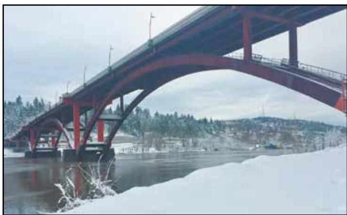
Winter snow covers the new Sellwood Bridge. According to officials the bridge is 99 percent complete. (Photo courtesy of Multnomah County)
