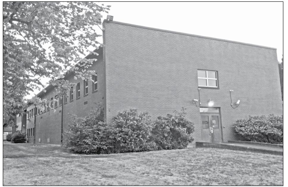
A fueling center is planned next to the former Sears Armory office building. (Post file photo by Erik Vidstrand)
