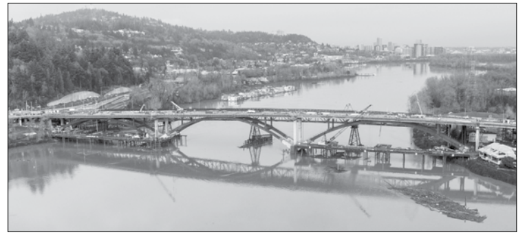
Aerial view of the new Sellwood Bridge as it appeared in January. (Photo courtesy of Multnomah County)
