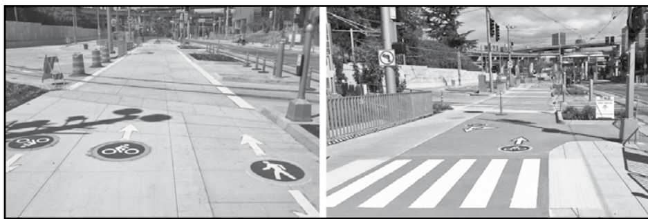
Pedestrian and bicyclist safety improvements along Moody Avenue in South Waterfront. (Photo courtesy of South Portland Business Association)
