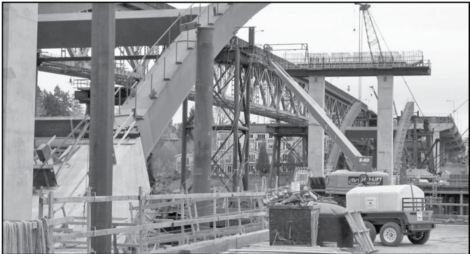
The east and center arch span segments on the new Sellwood Bridge are installed in sequence designed to load the weight evenly between the two spans. (Photo courtesy of Multnomah County)
