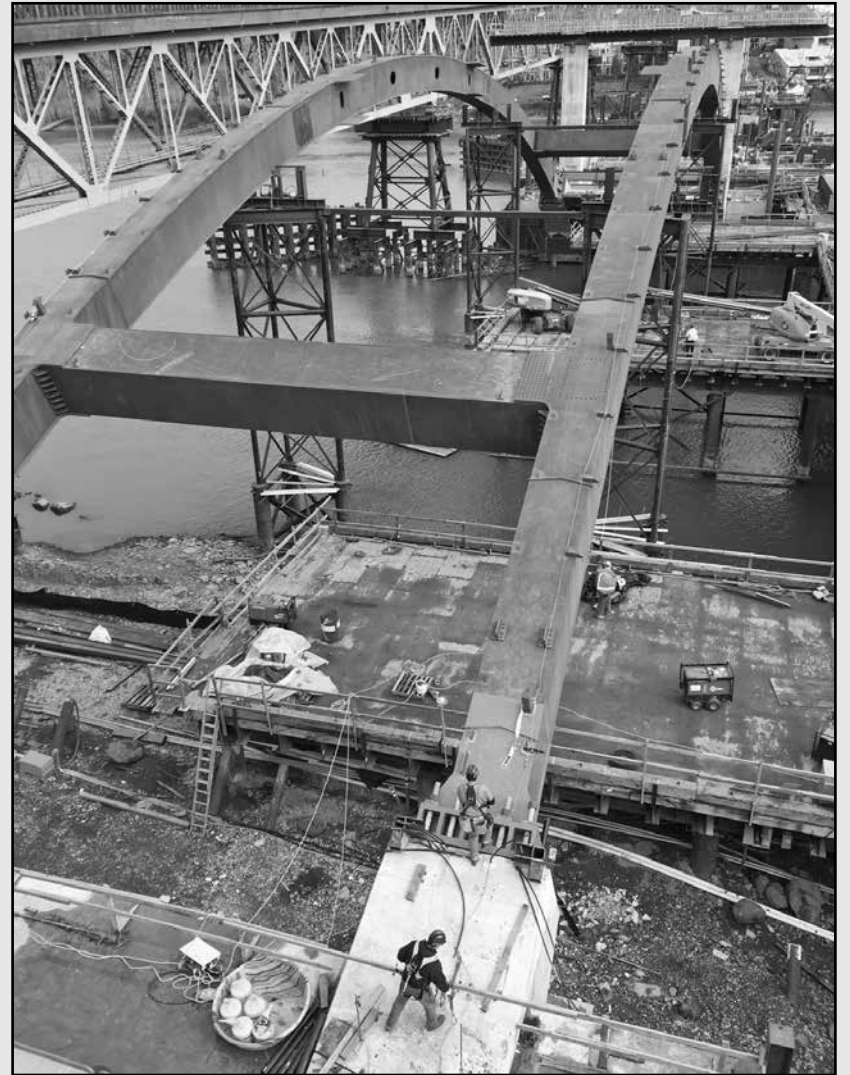
The contractor for the Sellwood Bridge continues to install cross braces between the two steel arches of Span 3, at the west end of the Sellwood Bridge. Workers are installing 3,000 bolts at each connection in the arch segments. (Photo courtesy of Multnomah County)
