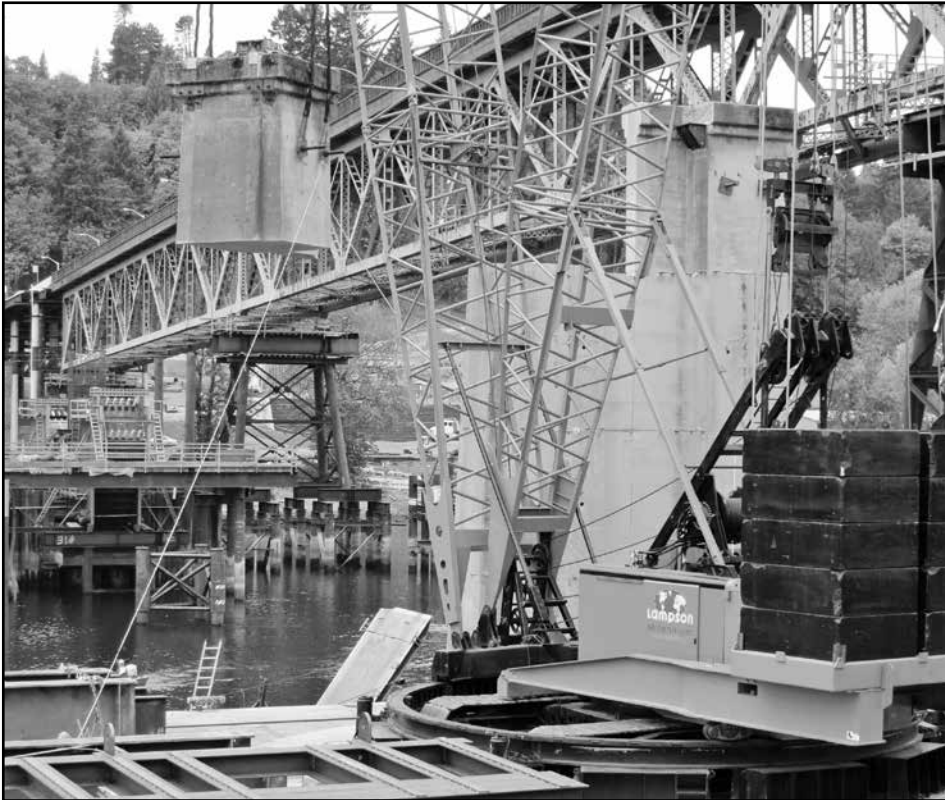
A crane removes a 300,000 lb. chunk of concrete from Pier 2. (Photo courtesy of Mike Pullen, Multnomah County)
