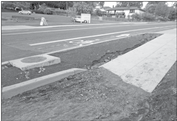
Mud covers the new sidewalk at the corner of Southwest 37th Avenue and Vermont Street after a two-hour cloudburst on Sept. 1. The ground is higher than the sidewalk in that area. (Photo courtesy of Rose Florek)
