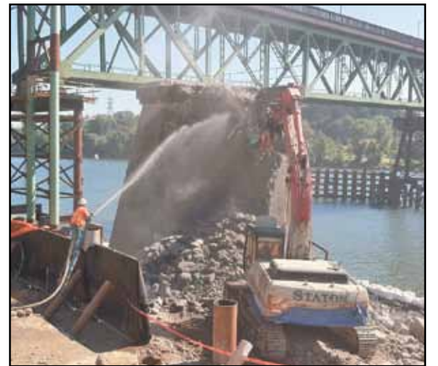
A Sellwood Bridge worker sprays a stream of water at one of the old west piers in July as a way to help control concrete dust during demolition. (Photo courtesy of Mike Pullen, Multnomah County)
