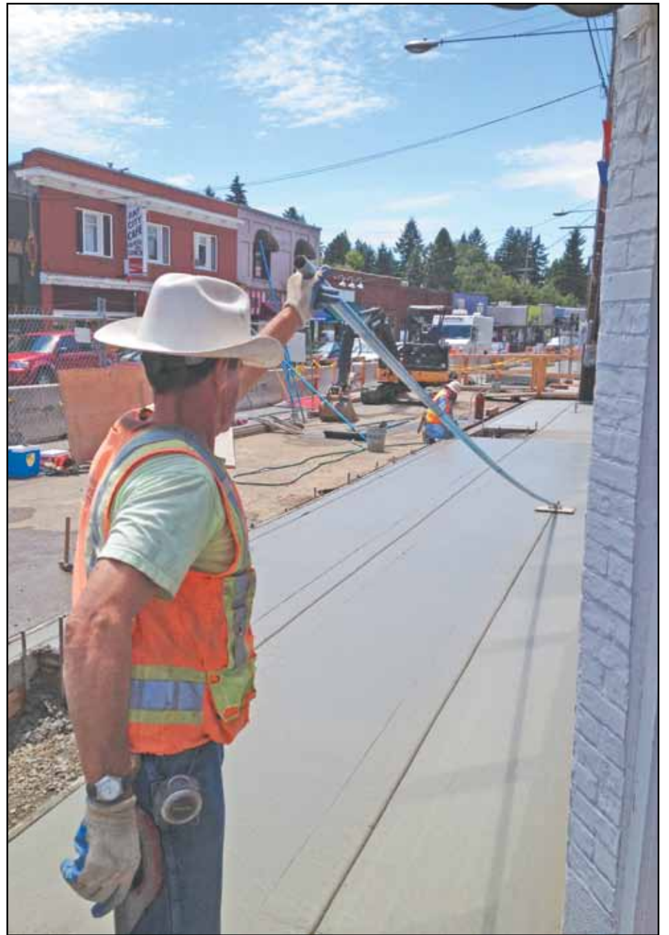
City contractors taking advantage of a dry day in June to pave one of the new sidewalks in the village. (Post photo by Erik Vidstrand)
