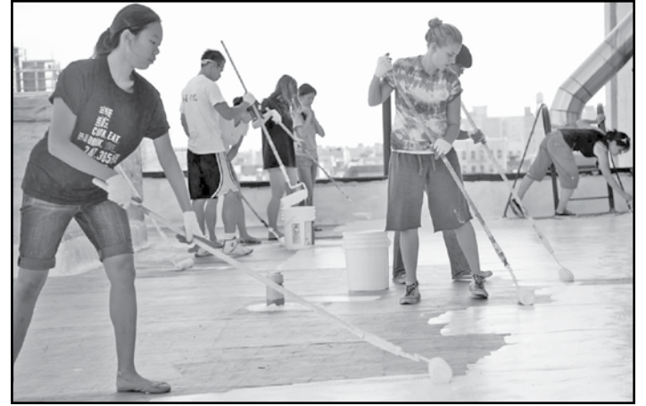
Some 90 percent of U.S. buildings have dark-colored roofs which, when exposed to full sun can increase in temperature by as much as 90 °F. A white roof typically increases temperatures only 10-25 °F above ambient air temperatures during the day. (Photo courtesy White Roof Project)
