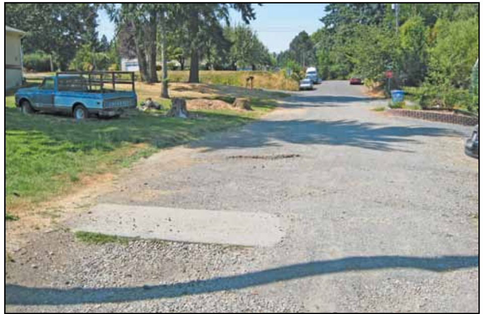
This is an example of one of the many unpaved streets in Southwest Portland. This is located close to 48th Avenue near Woods Park. (Post file photo by Leslie Baird)
