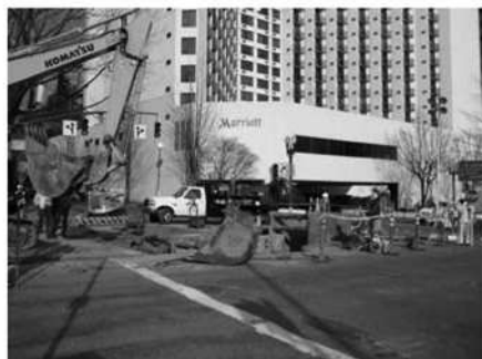
2007 work on SW Naito Pkwy at SW Clay St.
