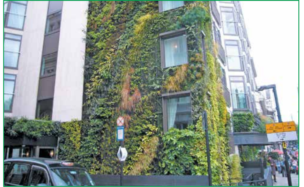
Green walls, or "vertical gardens," are walls partly composed of or filled in with live plant matter. They filter air and water, soak up carbon dioxide and help lessen the "heat island" effect of urban areas while reducing air conditioning costs in their host buildings. Pictured: a vertical garden at the Anataeum Hotel in London. (Photo courtesy of Niall Napier, Flickr)
