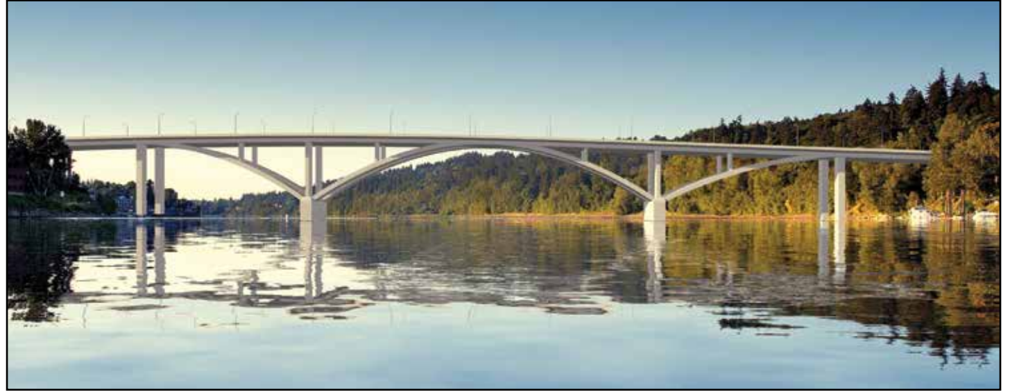
A photo simulation of a deck arch Sellwood Bridge replacement. (Photo courtesy of Multnomah County)
