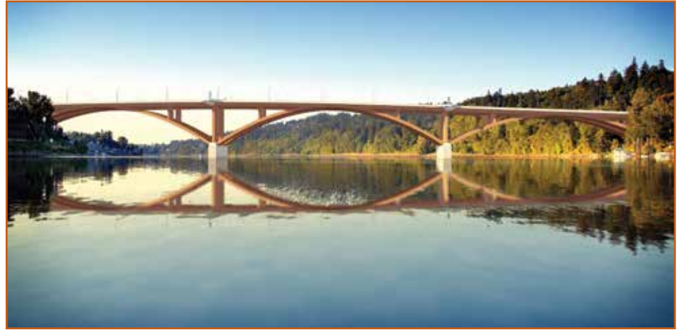
A new steel deck arch design (with the provision for using concrete if necessary) was approved by the Multnomah County Commission in January. (Photo courtesy of Multnomah County)
