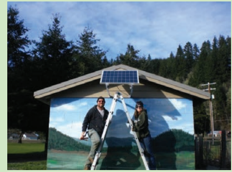
Alsea Community Effort, Alsea Emergency Power System
