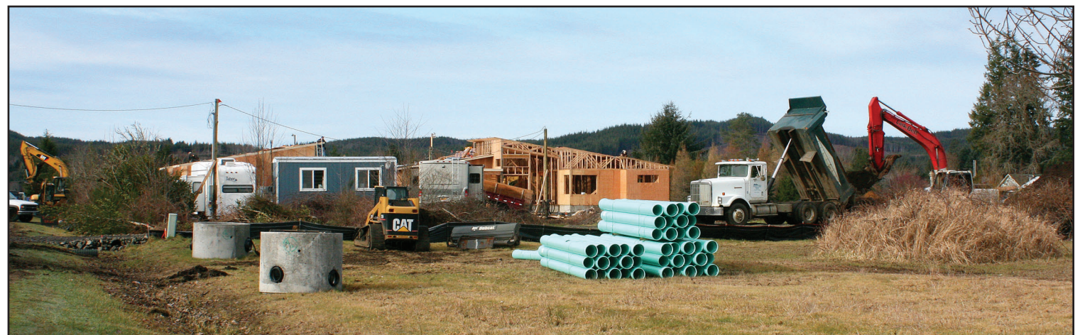
Housing and infrastructure construction continues at the Tillamook Community in Siletz.
