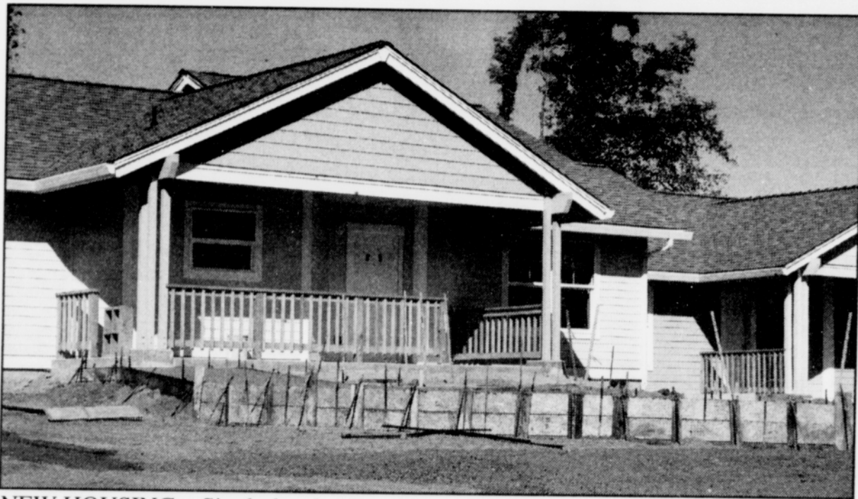
NEW HOUSING – Single-level units (above) and those in two-story buildings (right) near completion in early September. All units have a single-car garage, decks/porches with hand railings, forced-air furnaces, dishwashers, refrigerators and electric ranges.
