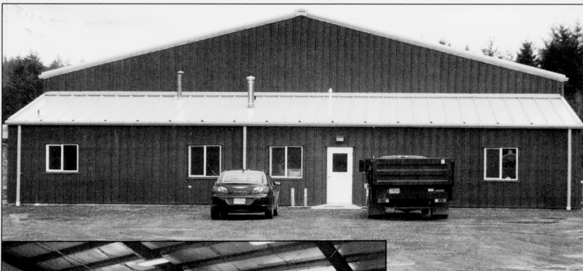
The new USDA building (left) nears completion in April, with a projected opening date in May. The inside of the warehouse area (below, left) is nearly ready to store food, as is the new freezer (left in photo). The nutrition education area (below) is almost ready to host cooking demonstrations. (photos by Diane Rodriguez)
