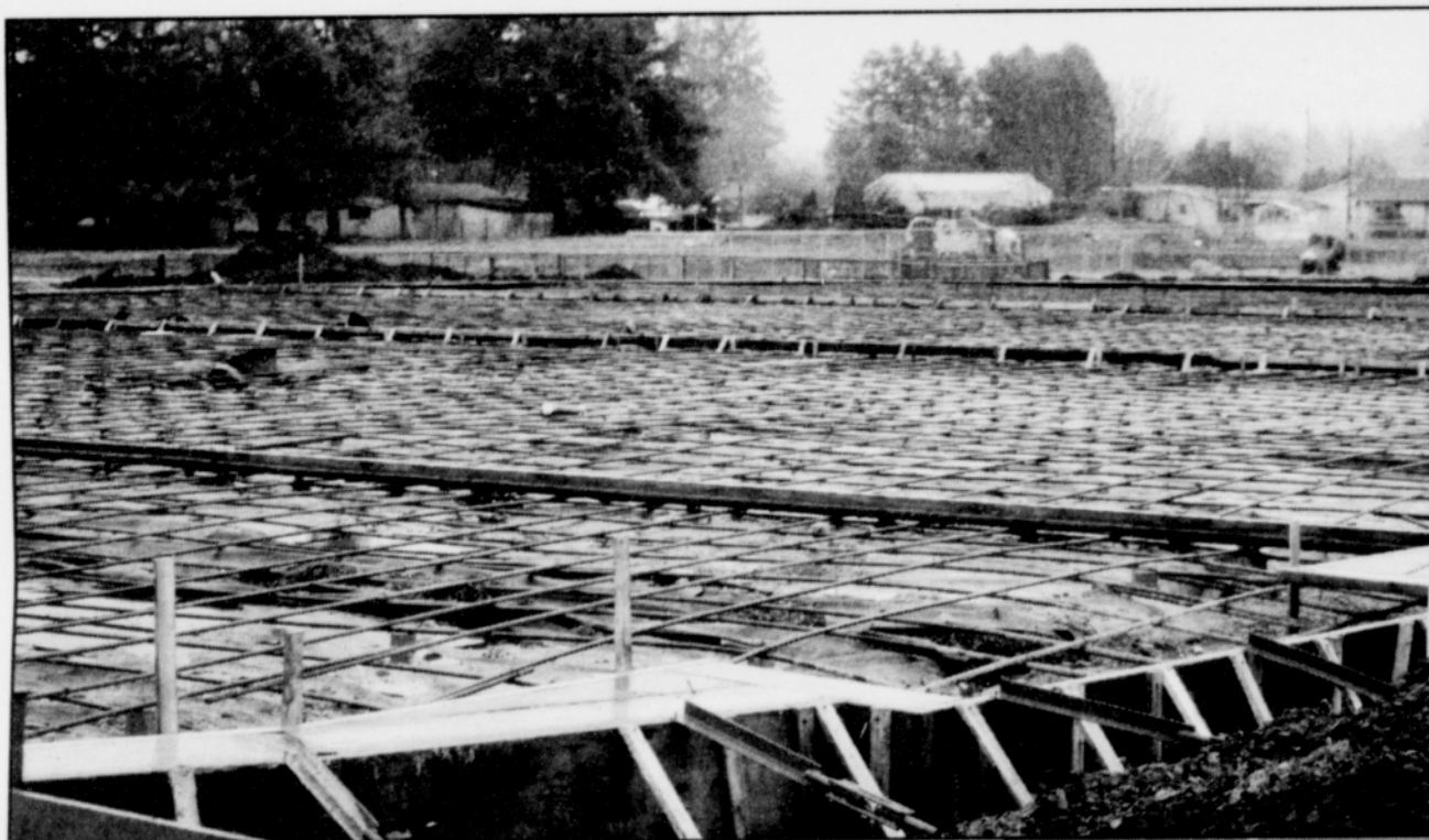
Left: The base of the cement pad for the Sprung Structure gym is completed and awaiting cement.
