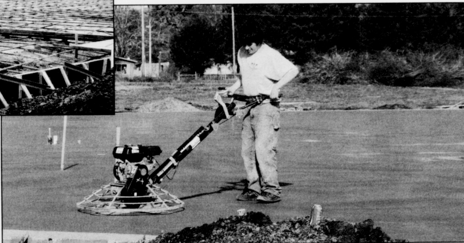
Right: The cement pad of the Sprung Structure gym receives finishing touches Feb. 15 as work progresses on constructing the new gym in Siletz.
