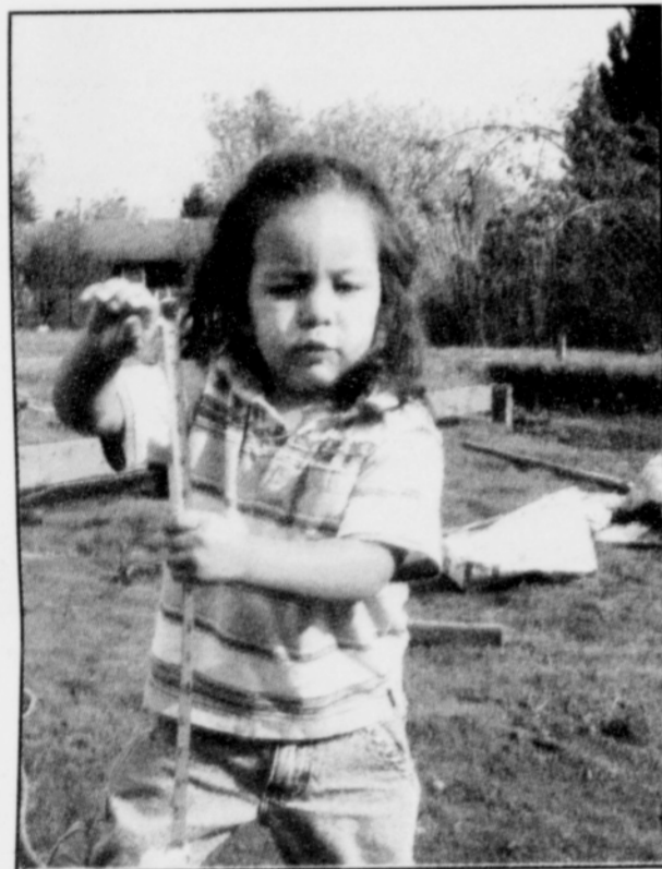
Lisa's grandson, Mossimo, helps with shop construction of the All Native Creations artists' co-op in Siletz.
