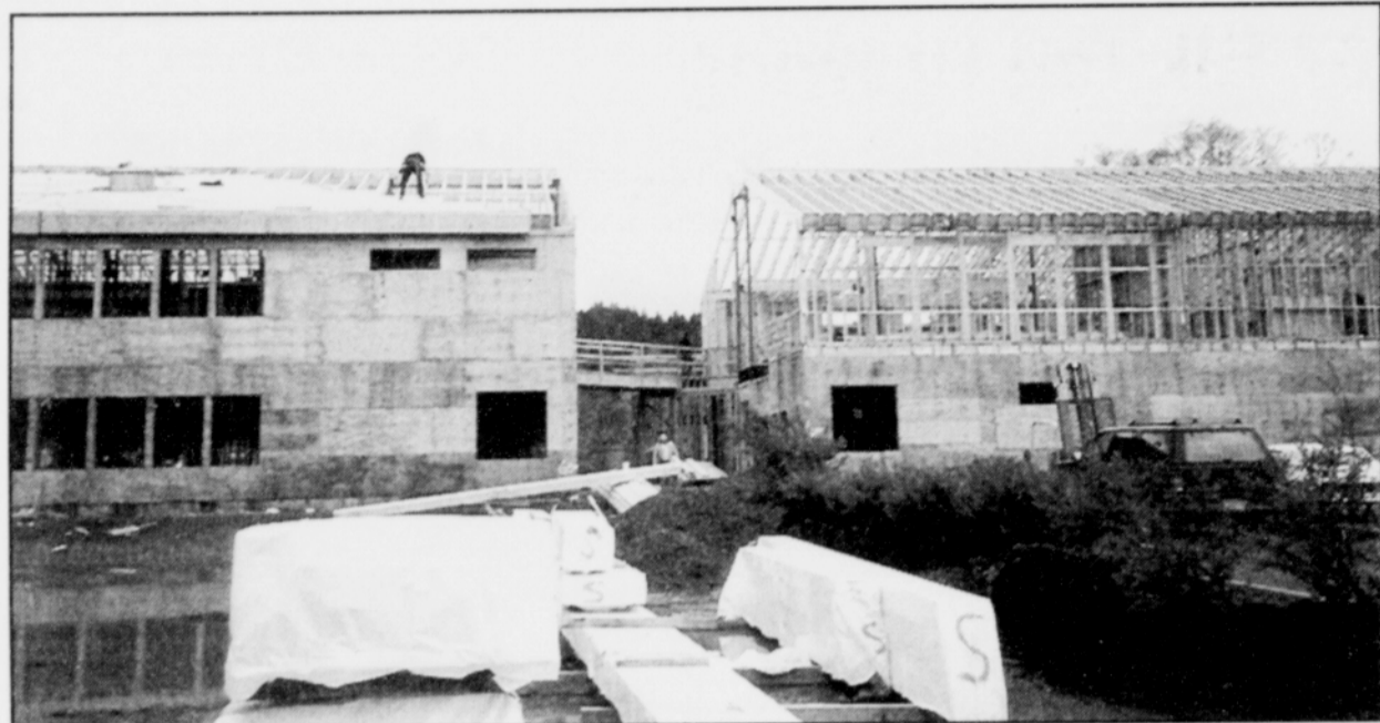
Construction progresses on the tribal administration building in the mid-1990s.
