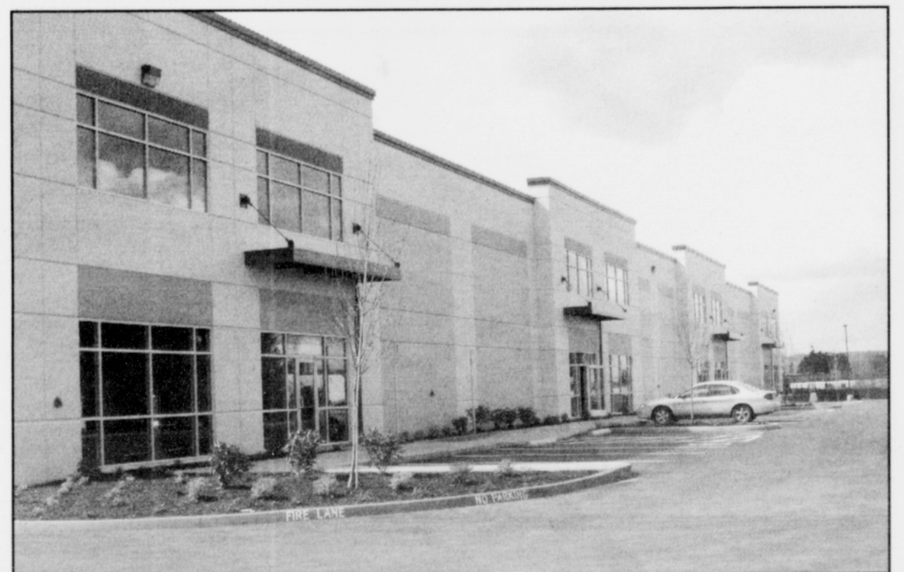
The front of the building that soon will house the Salem Area Office and the USDA food distribution warehouse.
