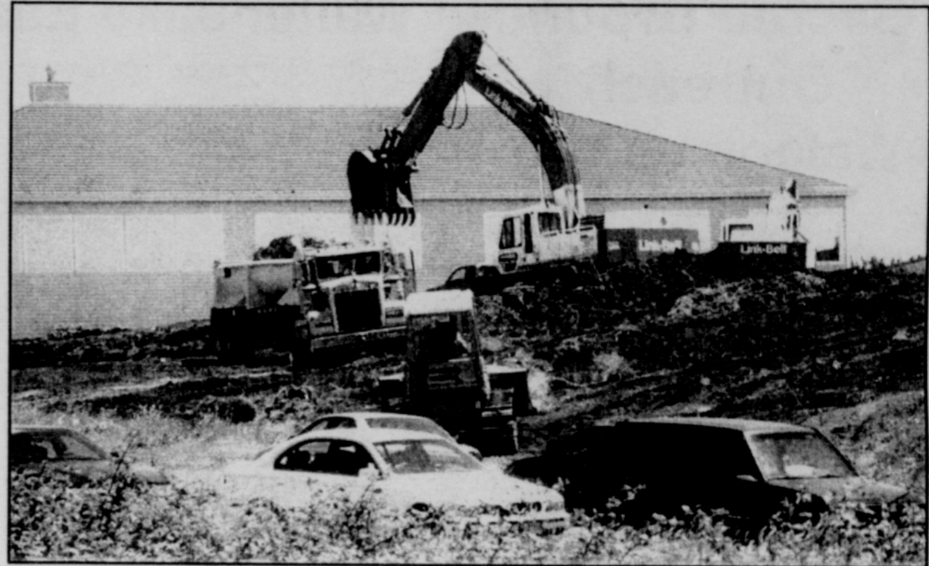
The parking lot expansion is under way.
