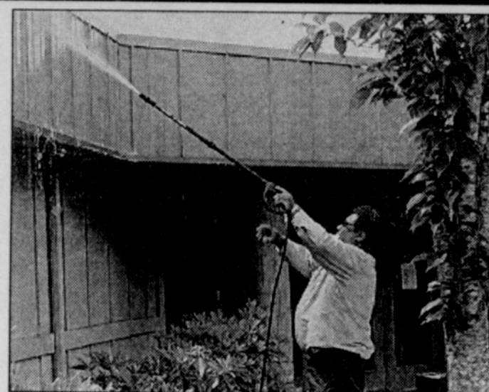
Bristo Bayya power washes the Siletz Community Health Clinic before the clinic receives a new paint job.
