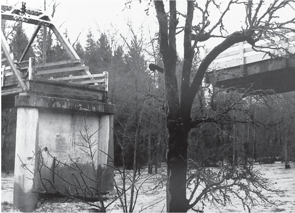
Flood-damaged Applegate Bridge in December 1955, near the mouth of Slate Creek. Photo: Josephine County Historical Society.
