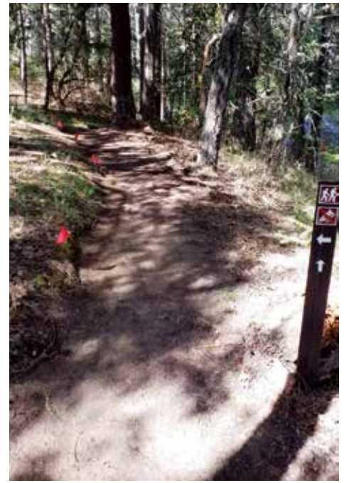
Ruch Community Outdoor School students have finished their work on this section of trail at Cantrall Buckley Park.
