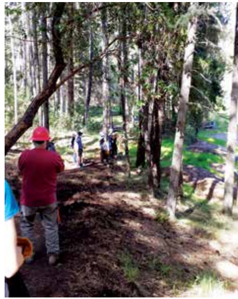
Students working on the trail after learning how to use the proper tools to angle the backslope, find the hinge point, and do the tread with a 3-5 percent outslope. The instructor, Duane Mallams (red hard hat), observes their progress.
