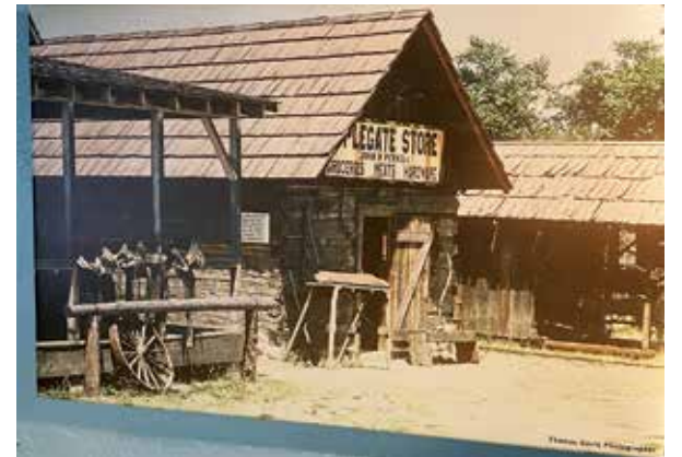
An early photo of the Applegater Store hangs in the current store. Photo: Michael Schneider.
