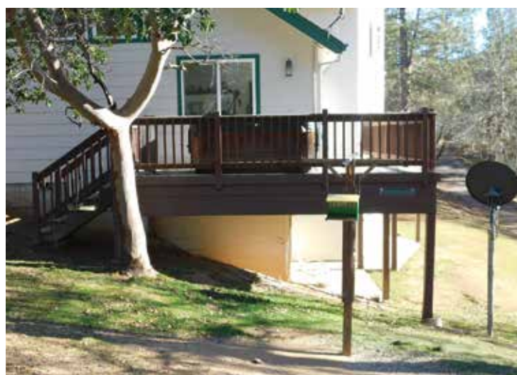
Keep spaces under decks and exterior staircases clean and free of dry vegetation. Sparks from a nearby fire could ignite leaves and the deck itself. Photo: Sandy Shaffer.
