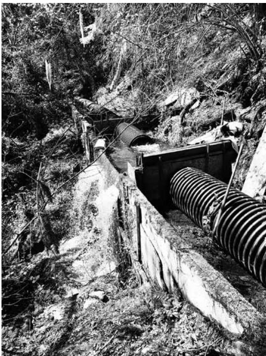
Weir located on the O'Brien ditch. The concrete work dates back to the 1930s. Photo: David Dobbs.
