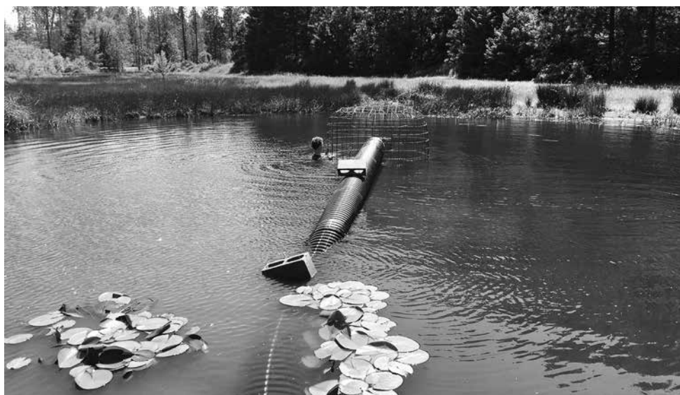
Jakob Shockey situates the cage before untying the float tube during a pond leveler installation. Photo: Timothy Sexauer.
