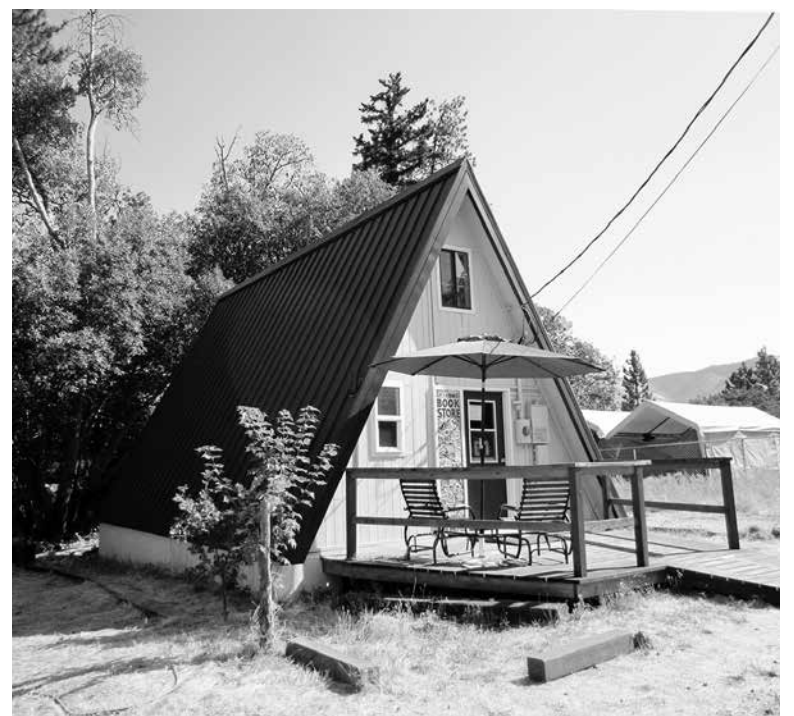
Check out the new roof on the FORL A-frame Bookstore, next door to Ruch Library.
