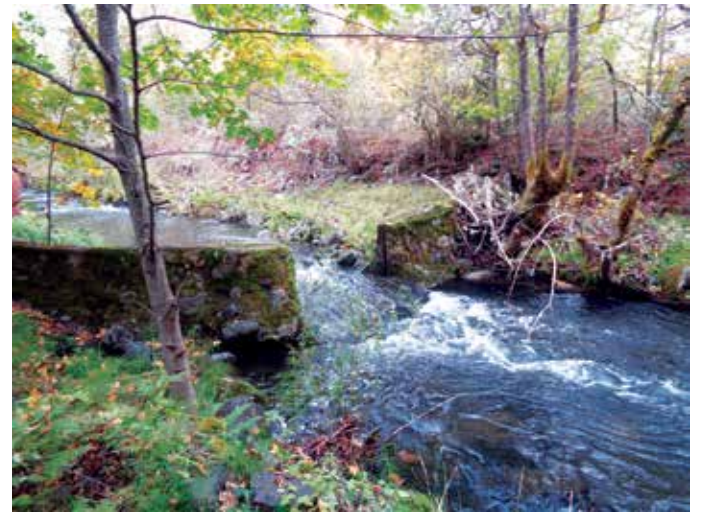
Now unused, this Powell Creek dam was historically used to create a pool for the landowner's tigers. Photo: APWC staff.
