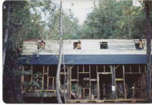
The "Big House" under construction at Molto Bene. Photo courtesy of Mike Kohn.
