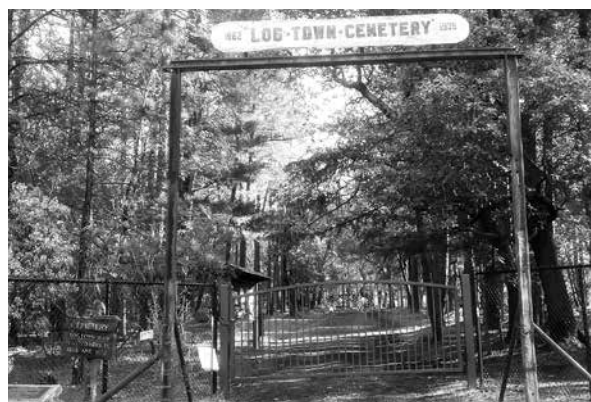
The wrought iron gate was made by Carl Offenbacher.
