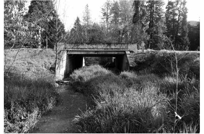
On Humbug Creek at the Highway 238 bridge, invasive reed canary grass was removed. With the help of Middle Rogue Steelheaders and Applegate School students, the streambank was stabilized and additional plants were added.
