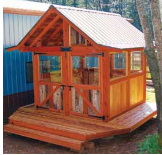
The Dragonfly Teahouse is made partially from reclaimed timber from the demolition of some Oregon mills.
