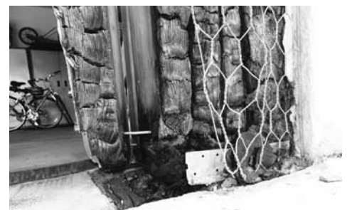
Interior ignition as shown here can be difficult for firefighters to spot during a wildfire. Above photos provided by Insurance Institute for Business & Home Safety.
