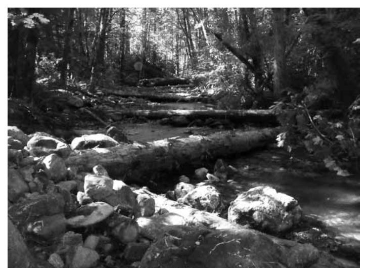
Over 90 logs were placed into the West Fork of Williams Creek to develop complex habitat reaches.
