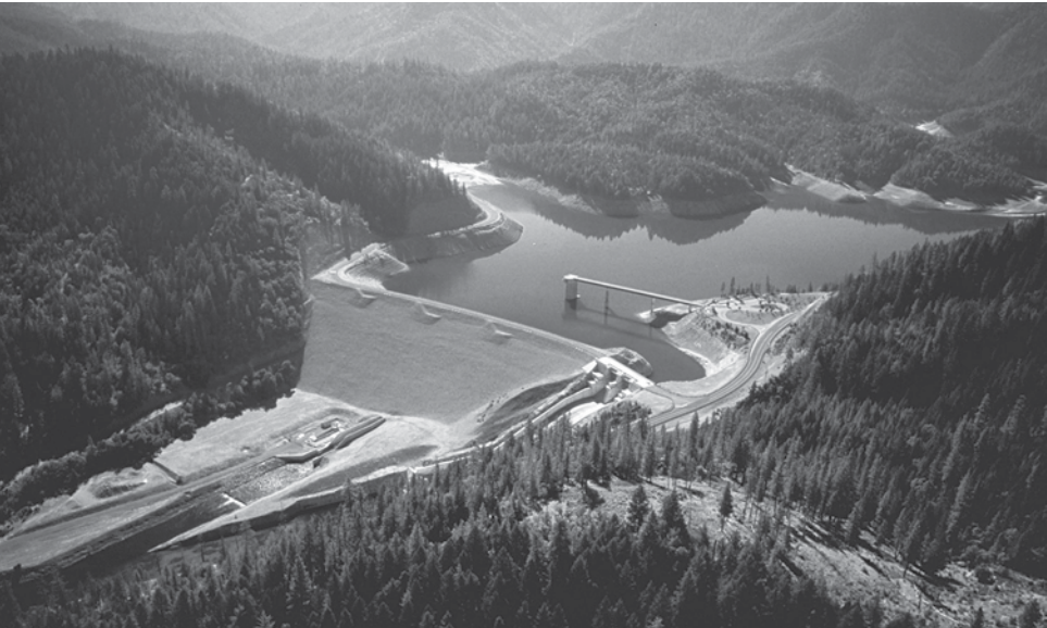
Applegate Dam looking south.
