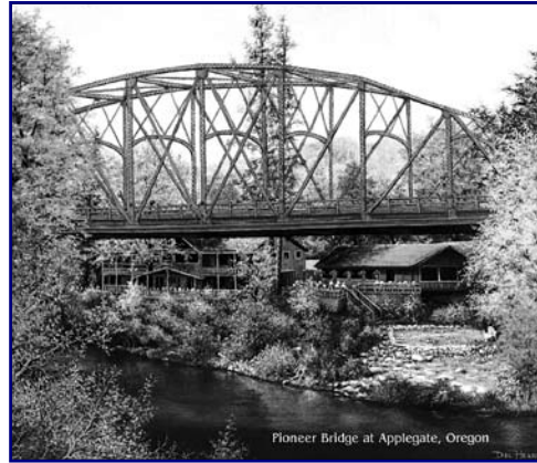
Pioneer Bridge at Applegate, Oregon
