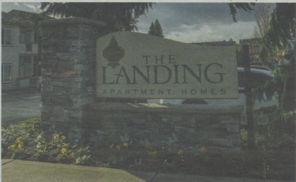
The Landing apartments are across from Oregon City High School off Beaver Creek Road nearly two miles by car and one for students to walk.
