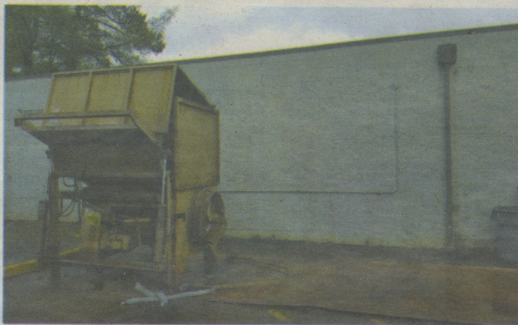
Bottom: The dumpster was removed, and the trash compactor was disconnected.
