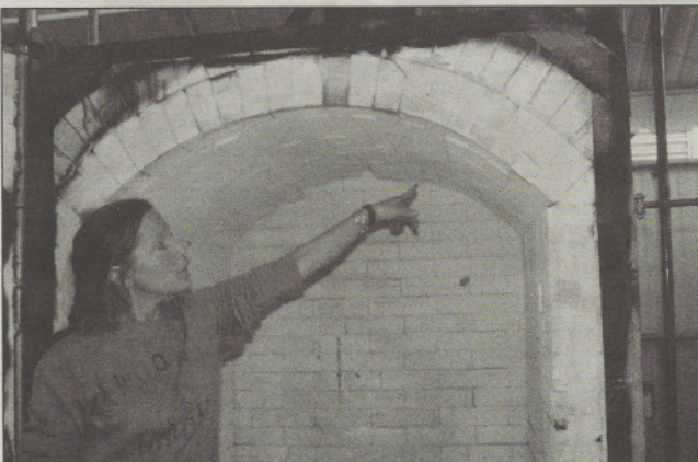
Kate Simmons points out the signs of age in the old kiln; loose bricks in the ceiling have begun to slide down and separate from the rest.
