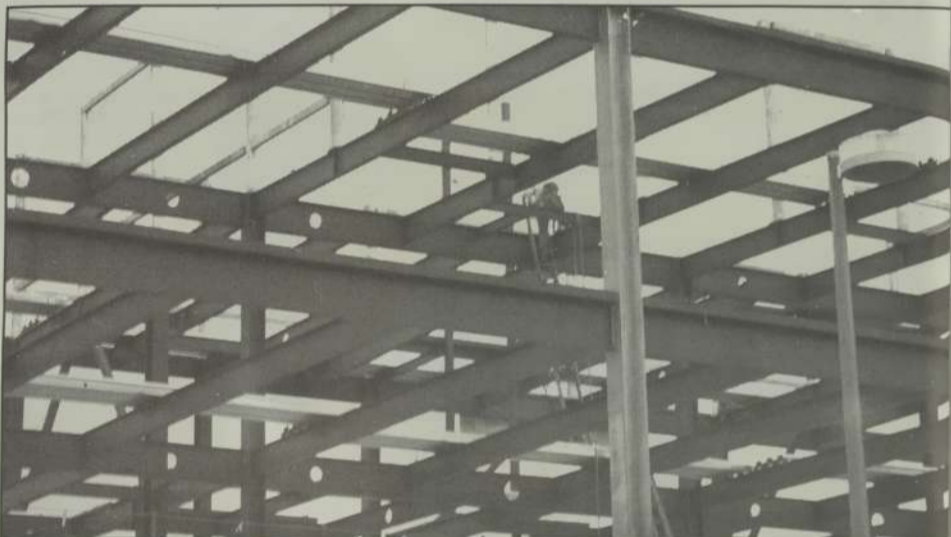
ABOVE: Builders continue work on the recent addition to Harmony Campus. BELOW: Structural steel is erected, serving as the backbone of the new building.
