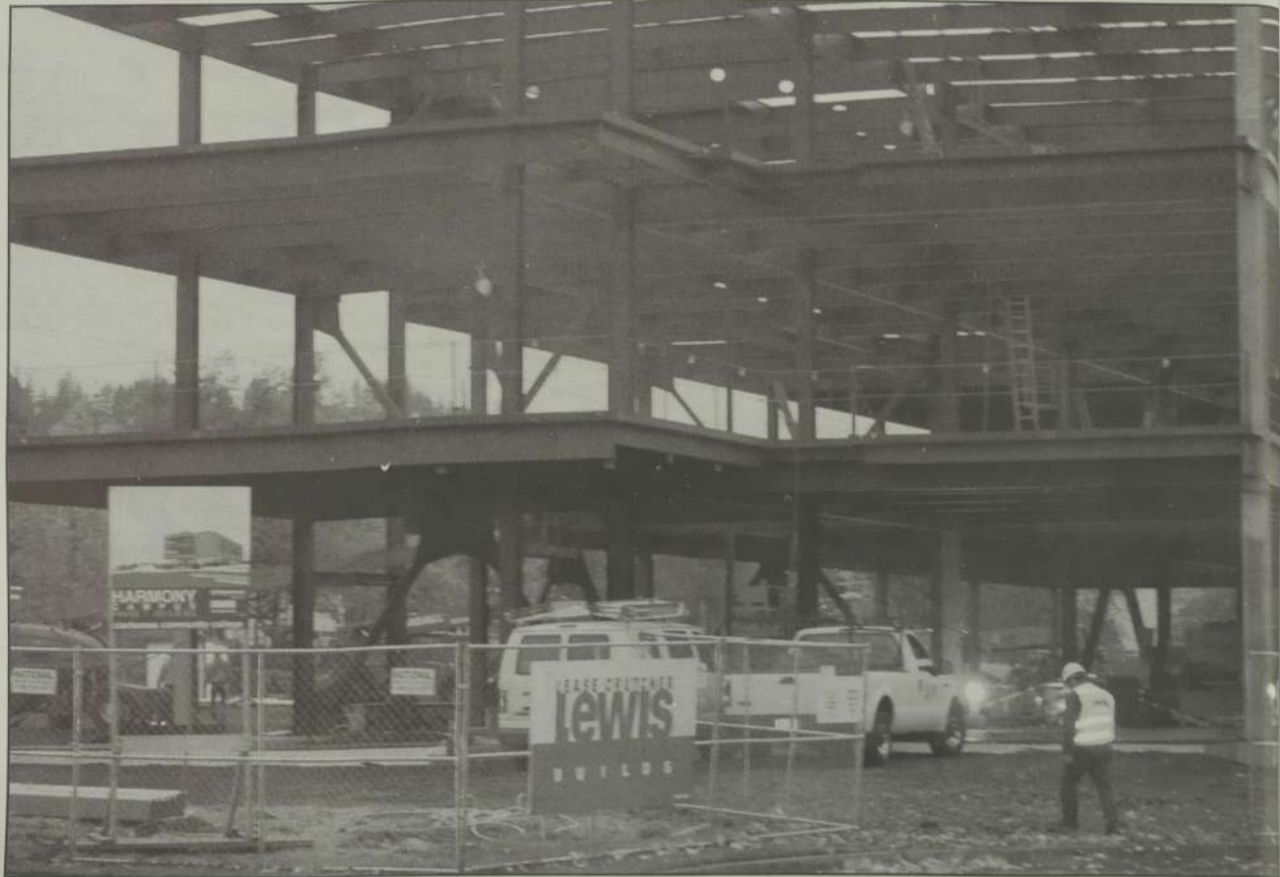
ABOVE: Builders continue work on the recent addition to Harmony Campus. BELOW: Structural steel is erected, serving as the backbone of the new building.
