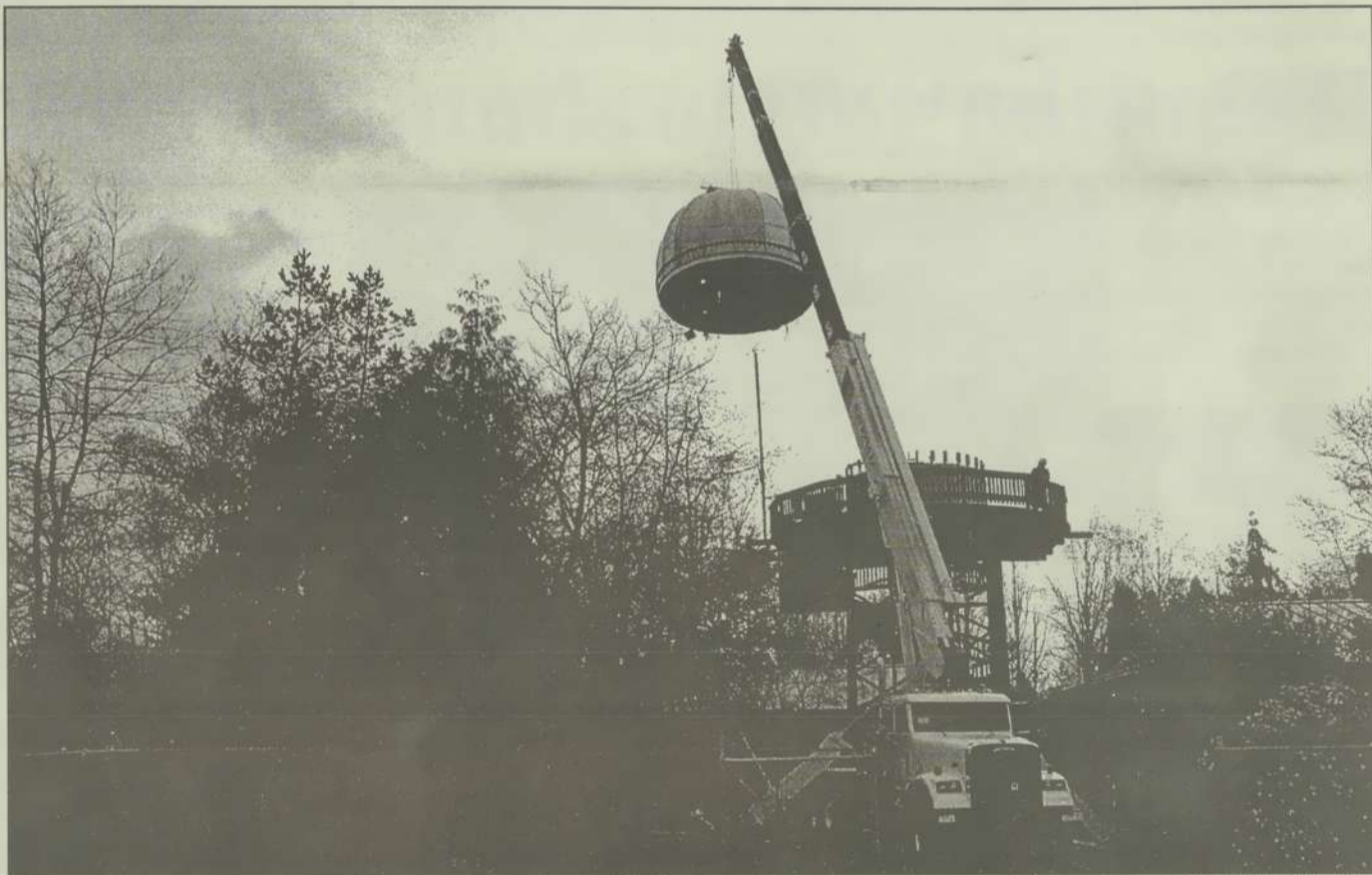
A crowd of twenty watched last Wednesday as the dome of the Haggart Observatory was removed for repairs. PHOTOS BY TIMOTHY A. BELL
